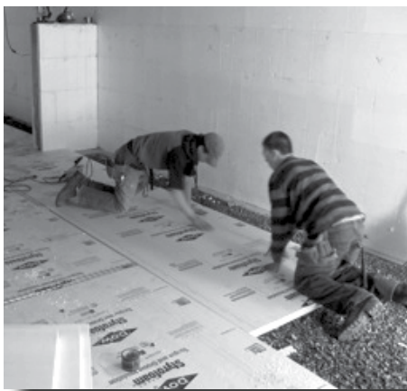
The students insulated the basement floor.
